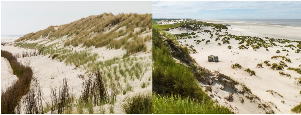
Figure 9. Left (A): Sand fences and marram planting on Ameland; Right (B): Artificially rejuvenated dunes on Terschelling (Photos: Alma de Groot).
