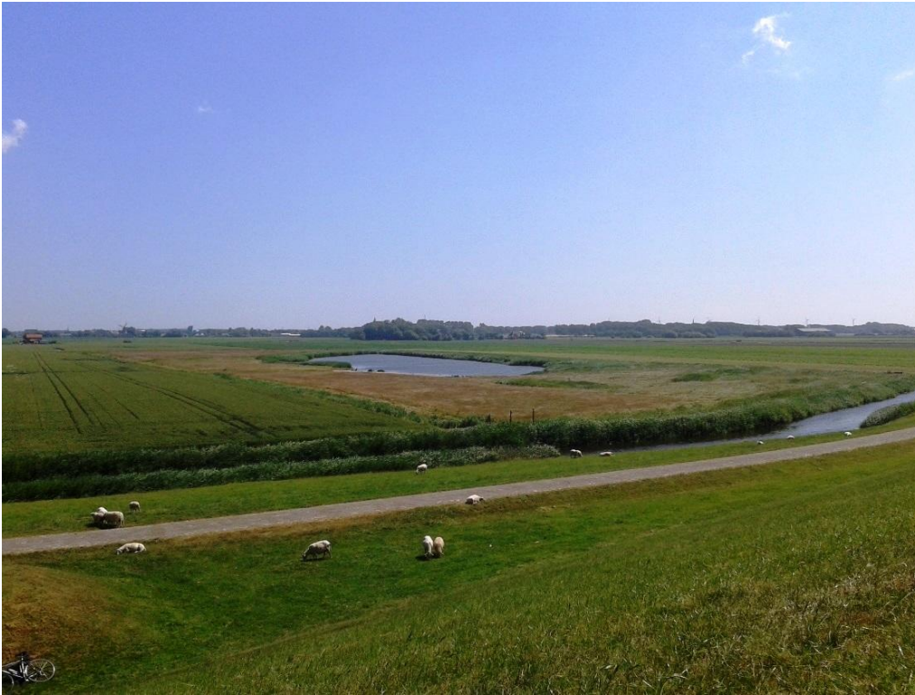
Figure 4. Wadden Sea dike near Sexbierum. The small lake is the result of clay-digging for dike heightening (photo: Meindert Schroor).
