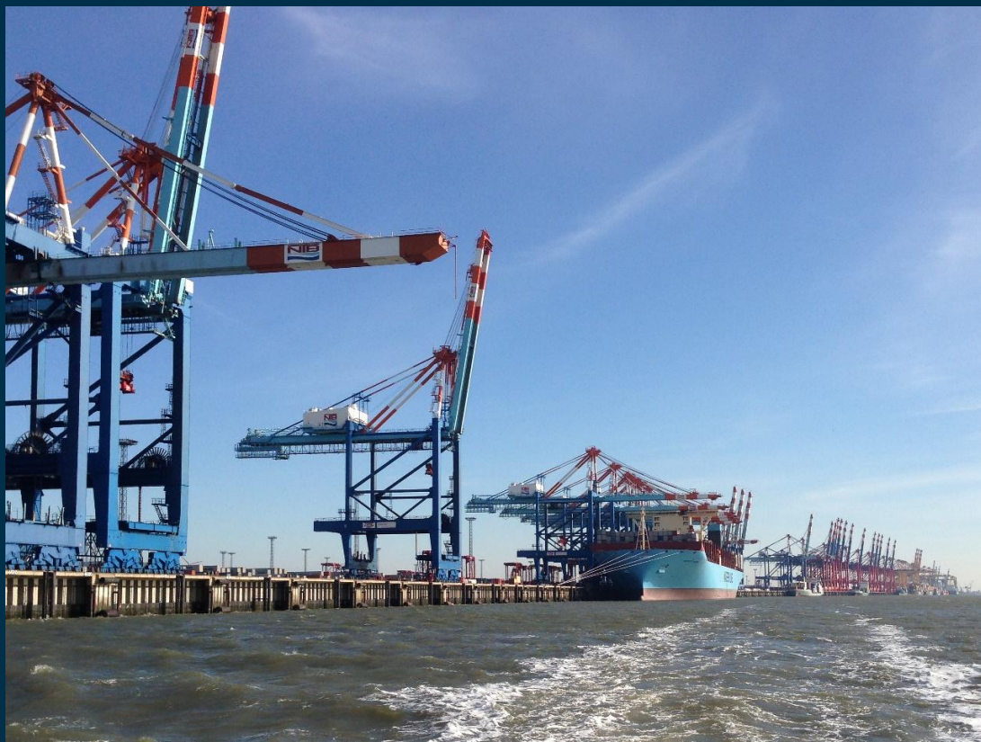
Photo: CWSS/ Bostelmann. Container terminal in Bremerhaven (DE).
